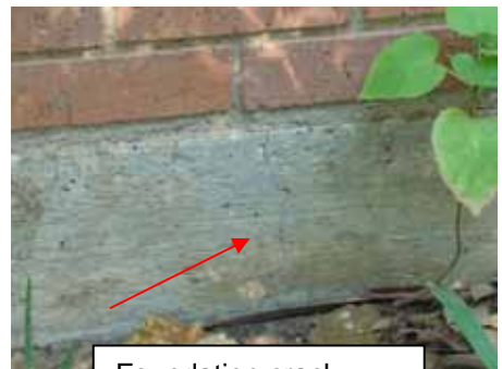
Foundation crack
