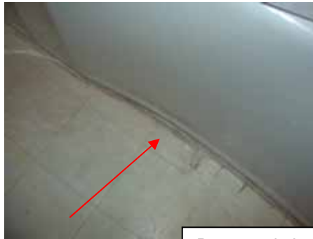
Damaged vinyl flooring
