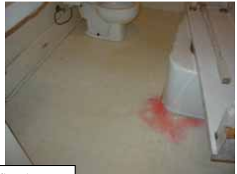
Damaged vinyl flooring
