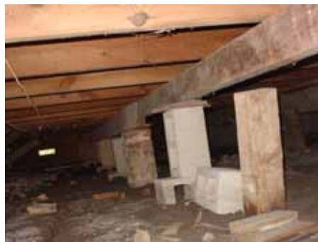
Beams are not properly supported.
